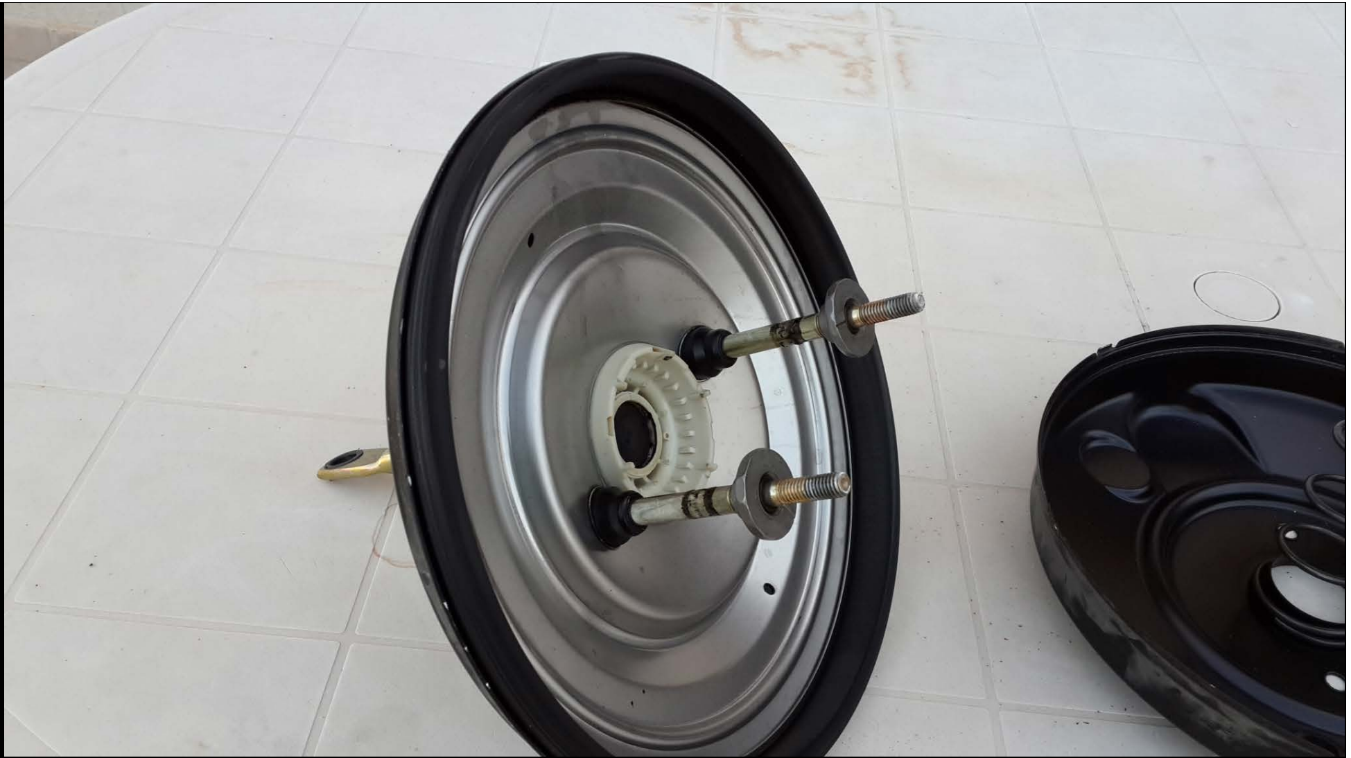
Leak was from that point.
