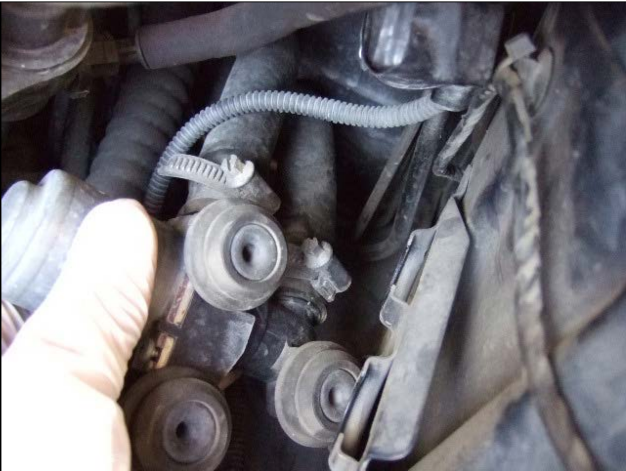
The new water valve Front:
